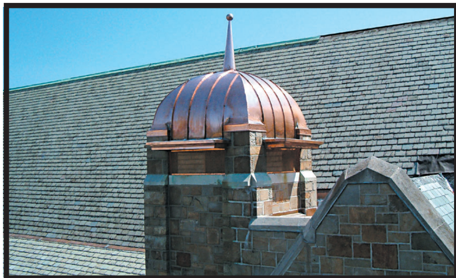
LDA Architects and Crocker Architectural Sheet Metal worked to restore the copper dome and slate roof repairs for the First Unitarian Society of Newton.
