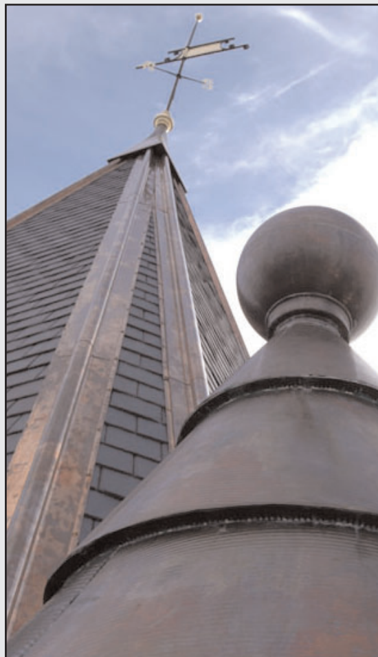
Exterior showing slate roof and copper flashing
