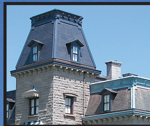
(Above) Restoration was recently halted as funds ran dry. Compare the historically accurate refurbished and restored tower to the deteriorated painted steel of the unfinished area to its right.
